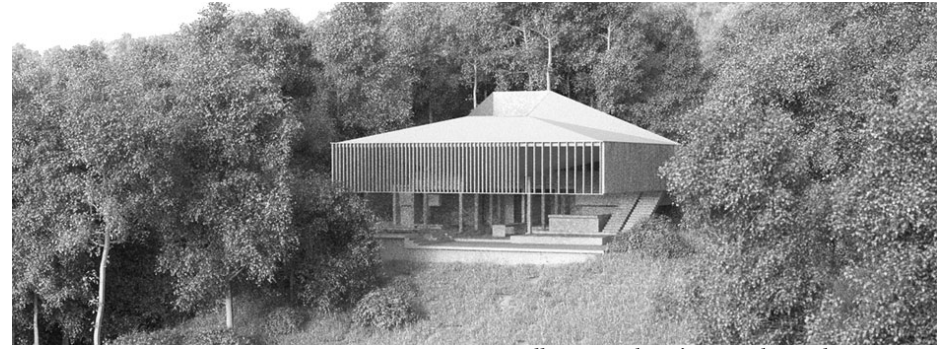
Williamson Chong's Fox Lake work in progress
